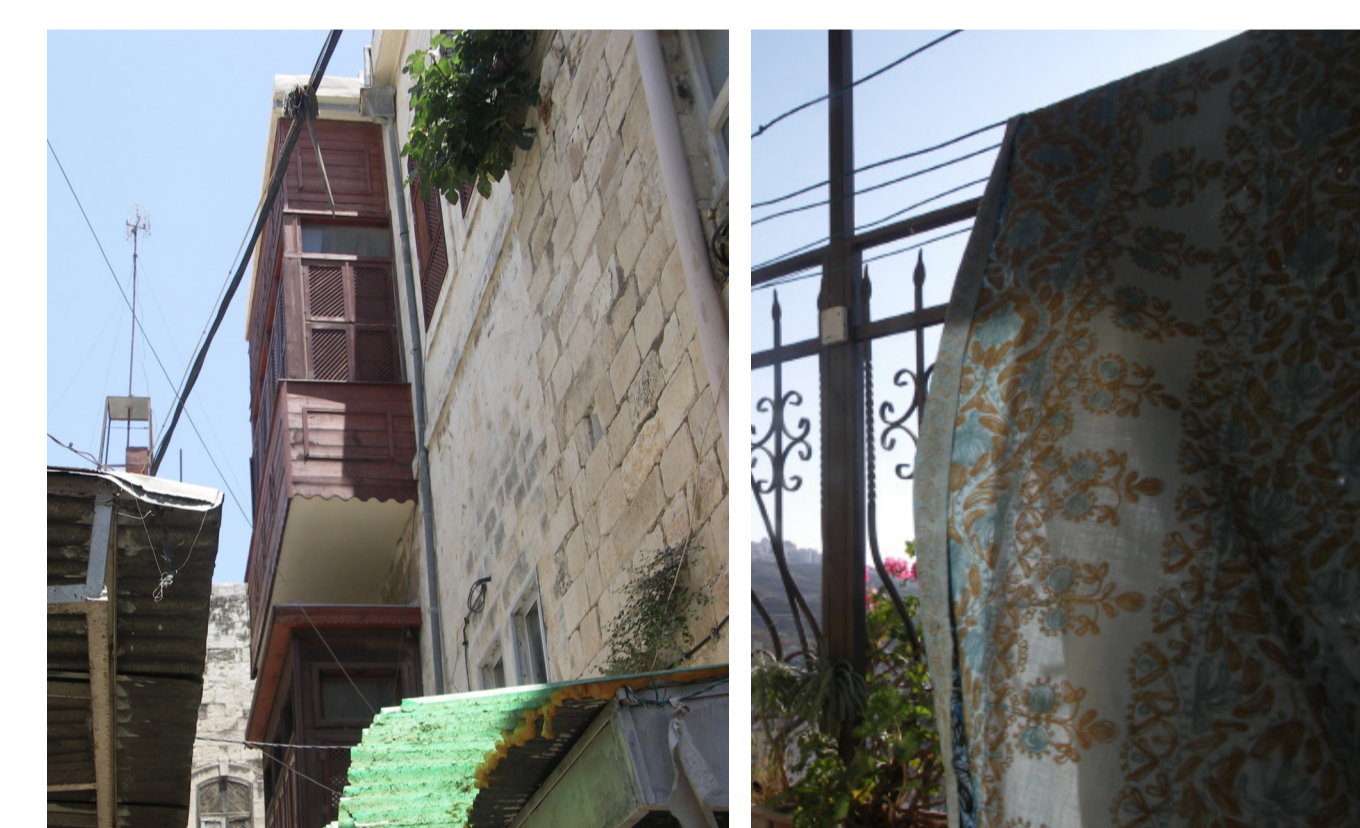
Figure 8: strategies to control natural lighting penetration: Traditional Moucharabiyeh (left), Modern fabric cloth (right)
