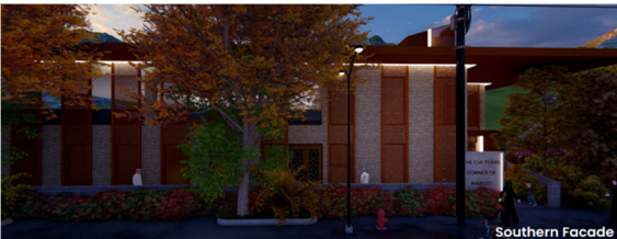
Figure 10. Decorative screens to reduce heat gain and allow for natural ventilation. By Aditya Chidananda, 2023.
