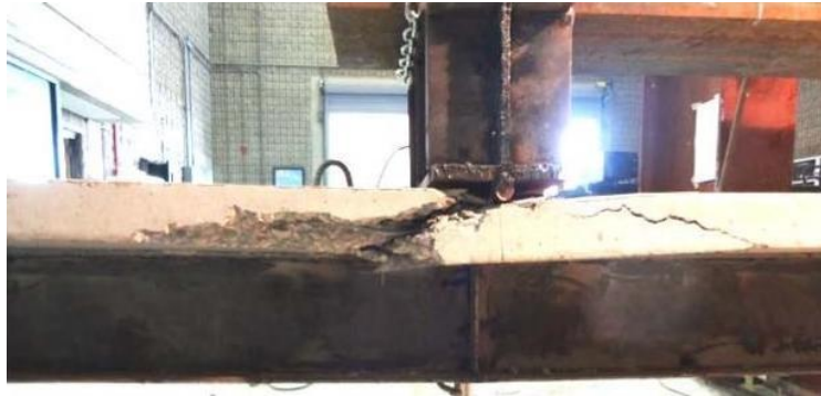
Fig. 14 Shear-compression failure at mid-span region
