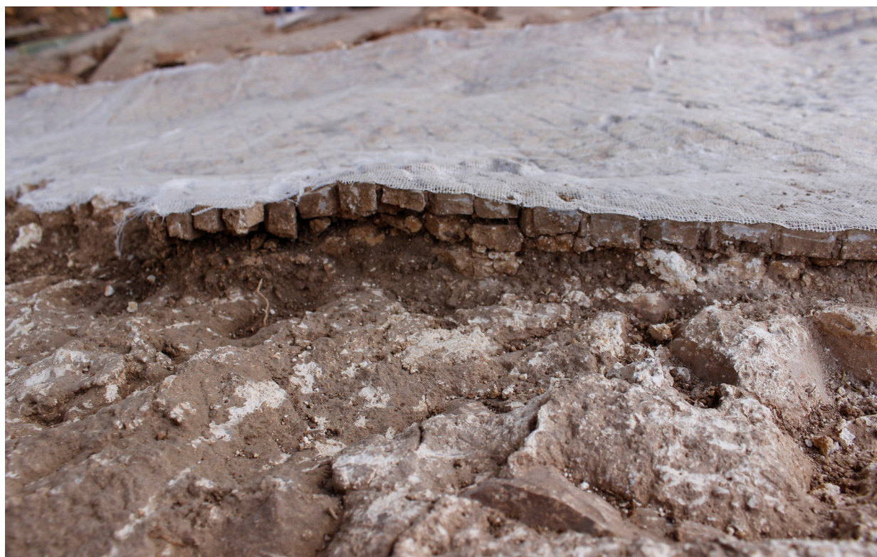
FIG. 9. The soil layer in between the bedding layer and nucleus in Room 3.
