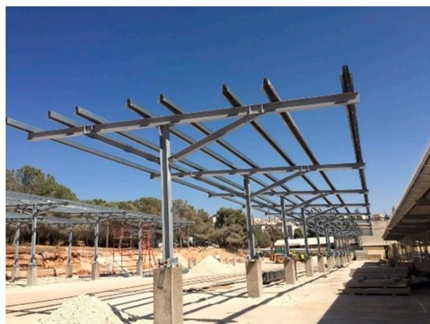
**Figure 1.** Steel-reinforced concrete anchors in solar-mounted structure.
