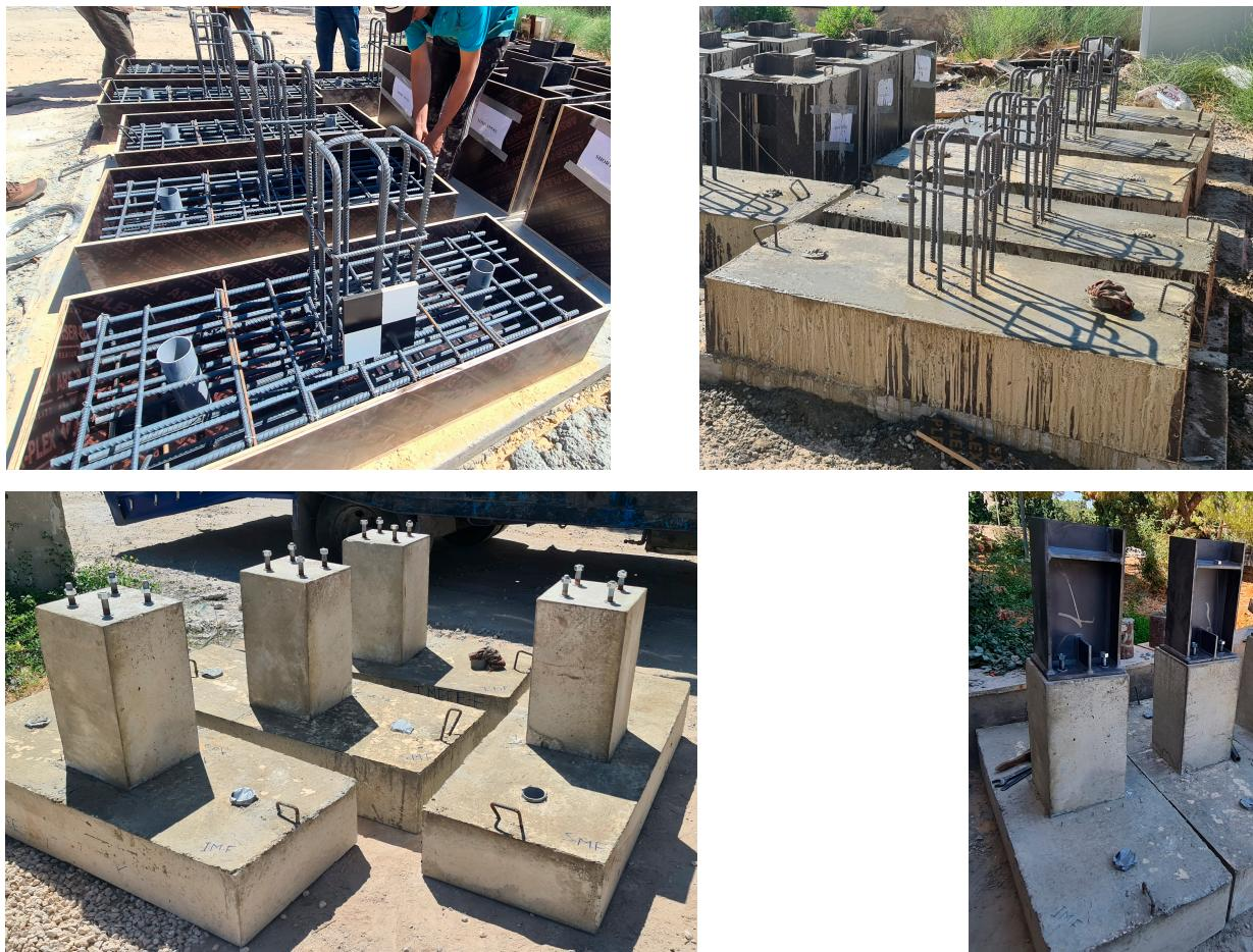
**Figure 4.** Photos of construction procedure of specimens.
