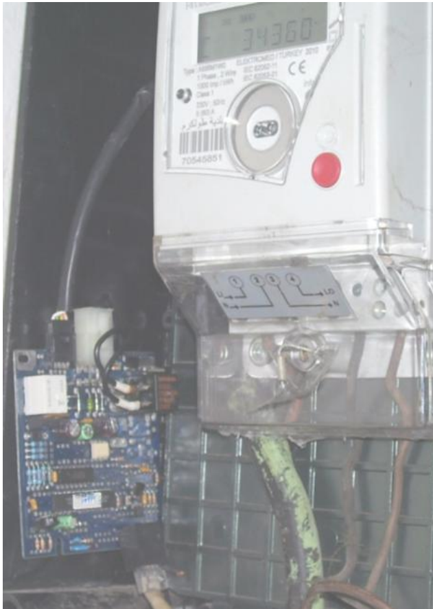
Fig. 3. ECU installation at the meter side
